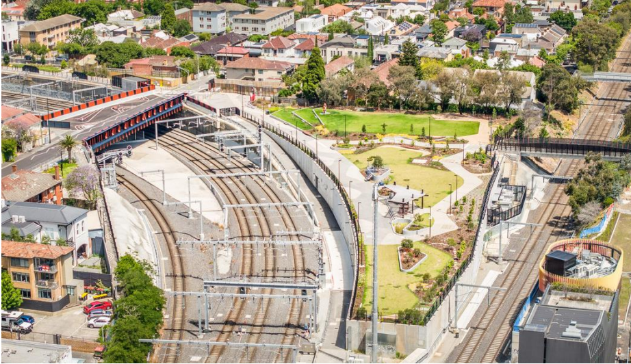
The new tunnel entrance including enhanced Siding Reserve, Lover's Walk, and Williams Street bridge.
